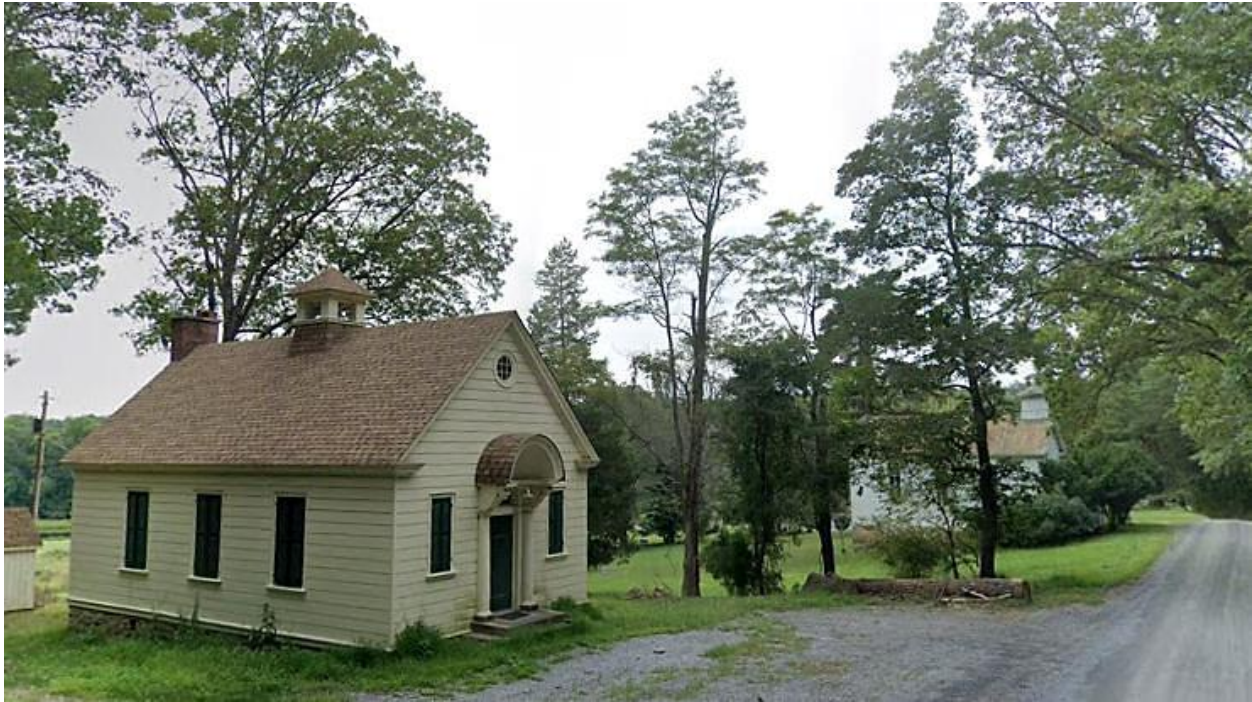
The Comstock School and Bell's Chapel of the Mt. Ephraim community in Frederick County, MD. These buildings illustrate some of the important institutions for Black communities after the Civil War. (Google Maps Street View, 2019)
